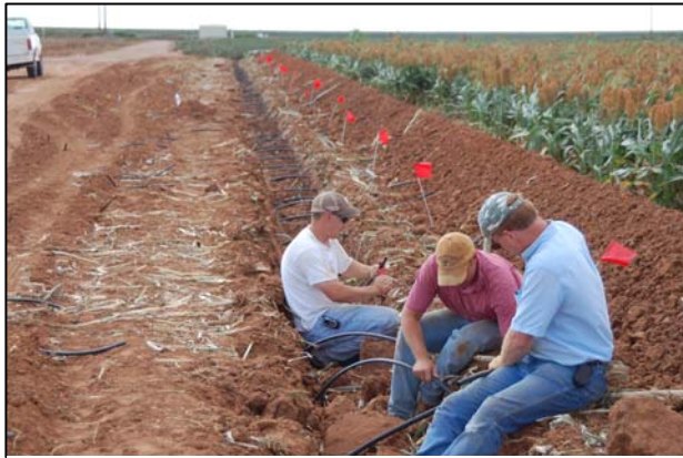
Reinstallation of SDI laterals. Previous work on SDI design had been complete and new SDI laterals were installed for future experiments, Helms Farm, 2007.
