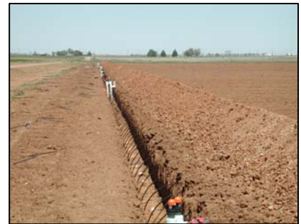
Figure 1. Drip tape installation.
