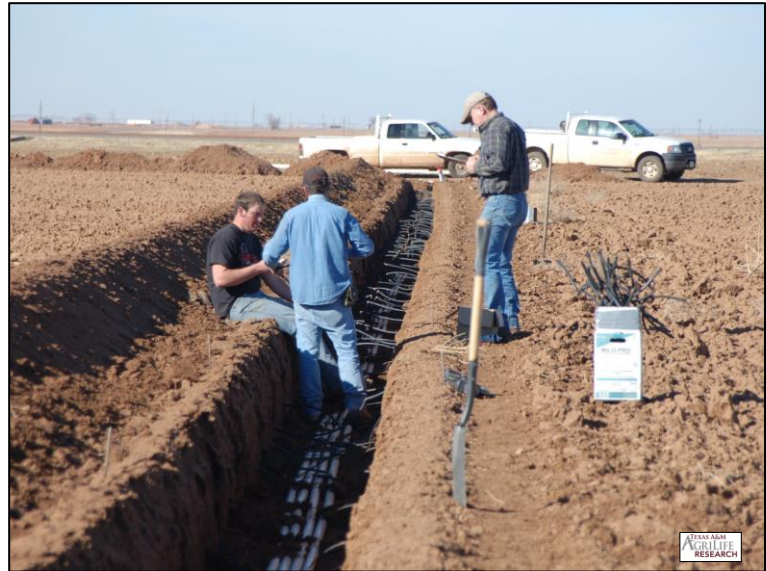
Figure 1. Installation of subsurface drip irrigation for experiments at the Helm Research Farm, Halfway, TX.
